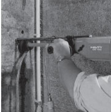
Press the core bit through the water collector (sealing disc, centering ring) onto the surface to be drilled. Switch on the DD 100 by pressing the main switch.
